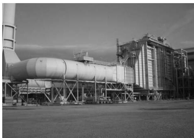
Figure 10 Group 4 stage 4-1 HRSG, exhaust duct
