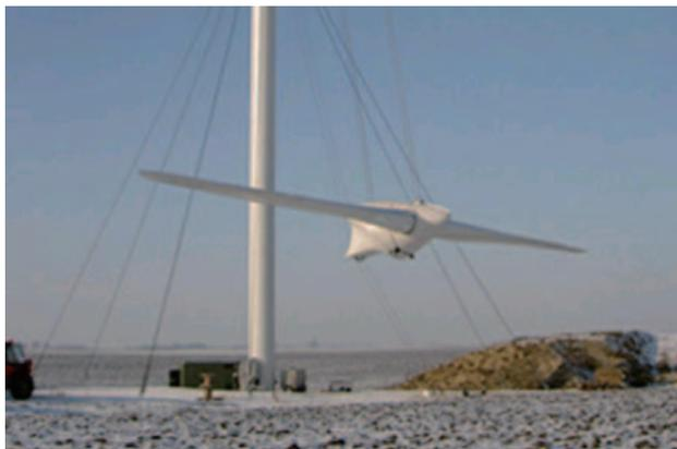
図6 Vergnet GEV HP-1MW施工状況<sup>11)</sup>
