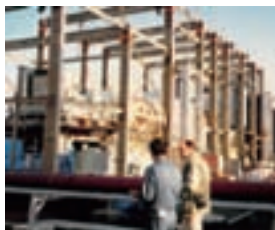
3 rd -1983, at TEPCO - Sodegaura Station: 100MW Reheat Gas Turbine, (AGTJ 100A in Moonlight Project)
