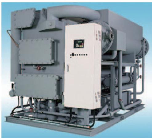
Fig.12 Steam driven absorption refrigerating machine
