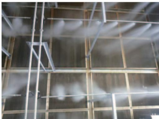
Fig.16 Nozzles of unadjusted angle (straight, downstream)
