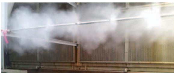
Fig.17 Nozzles of adjusted angle (upstream)
