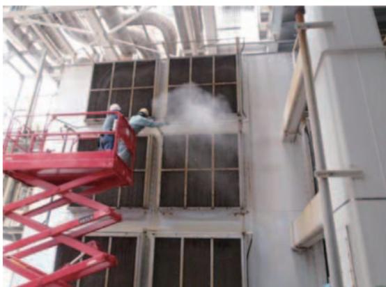
Fig. 12 Adjustment of nozzle angle at each section
