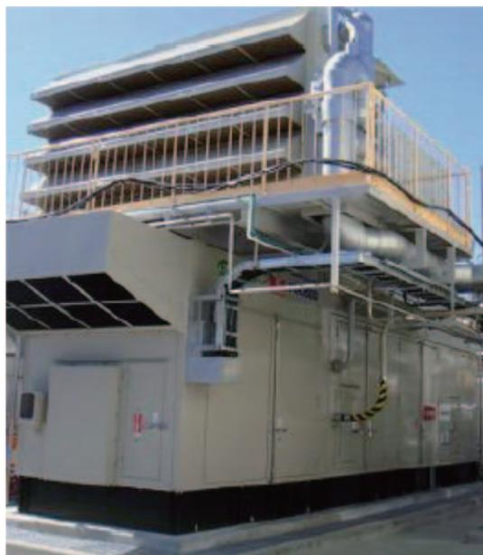
Fig.13 Cooling water inlet cooling system for PUC80D
