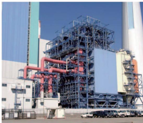
Fig. 7 De-sulfurization system of Isogo #1
