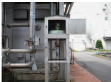
Fig. 8 Additional oil mist fan
