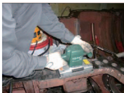
Fig.20 Improvement of assemble work by electrical operation
