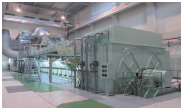
Fig. 4 Ishigaki No.2 power plant (diesel generator)
