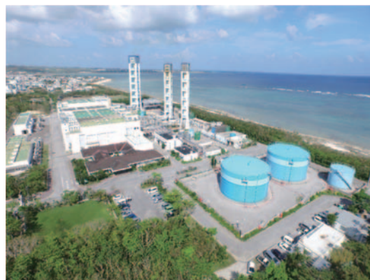
Fig. 3 Ishigaki No.2 power plant
