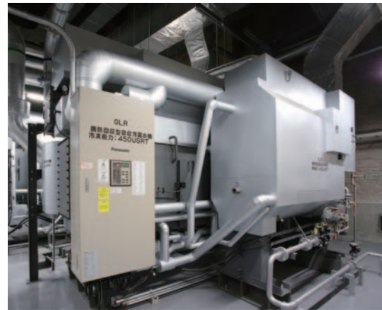
Fig. 7 Heat recovery absorption chiller (Hot water utilization)
