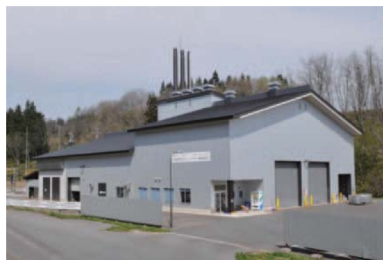
Fig. 1 External appearance of biomass power plant
