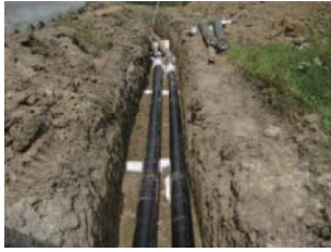
Fig. 11 Hot water piping distribution
