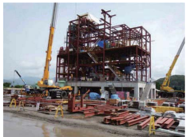
Fig. 3 Boiler under construction in 2014
