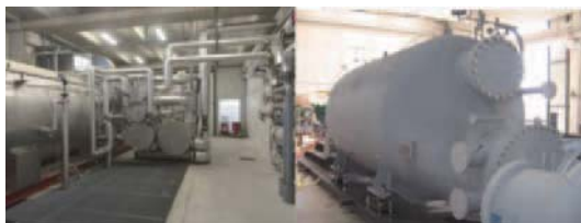
Fig. 13 Outline of Heat exchangers
