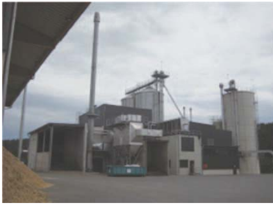
Fig. 19 Plant view of 0.8MW CHP
