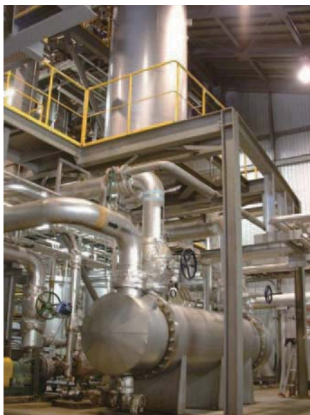
Fig. 13 Tar treatment equipment
