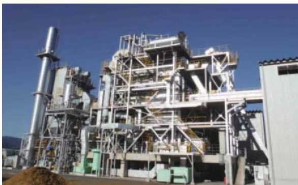
Fig. 1 Sukumo Biomass Power Plant
