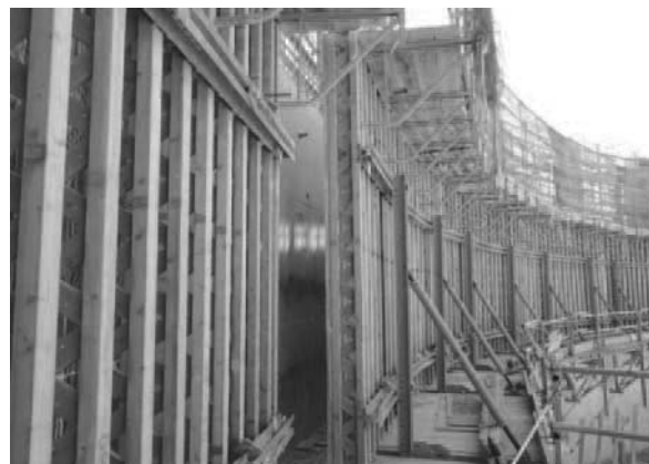
Fig. 4 Formwork and scaffolding system
