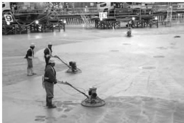
Fig. 5 Surface leveling of placed concrete
