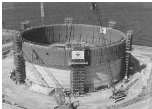
Fig. 3 Jumping form method of outer wall at Senboku, Japan
