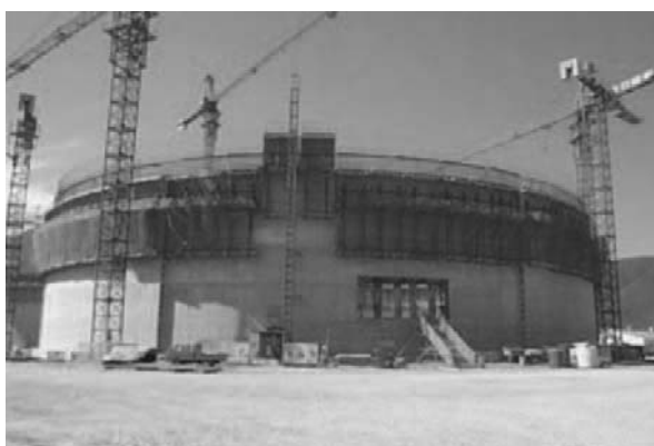
Fig. 5 Jumping form method of outer wall in Korea
