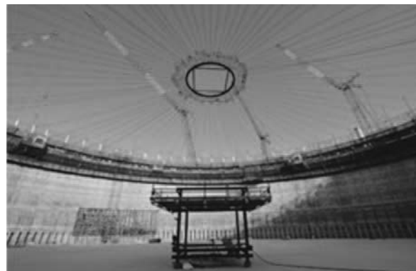
Fig. 12 Spoke wires (the adjustment mechanism)
