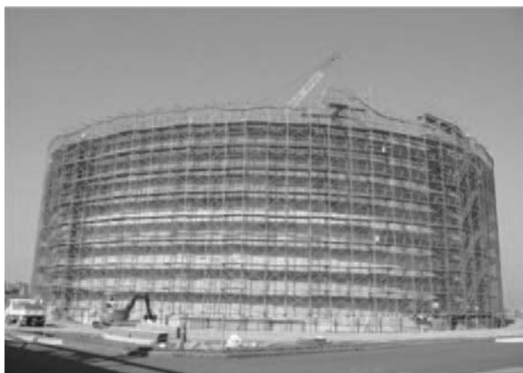
Fig. 2 Full scaffold method in Japan
