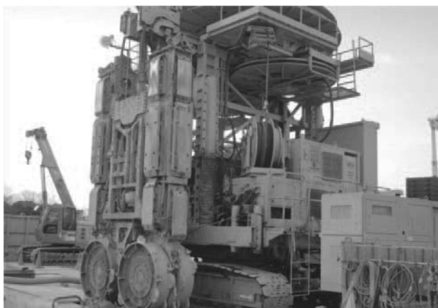
Fig. 8 Excavator of slurry wall
