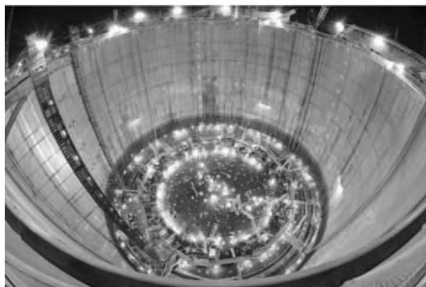
Fig. 7 Cylindrical slurry wall
