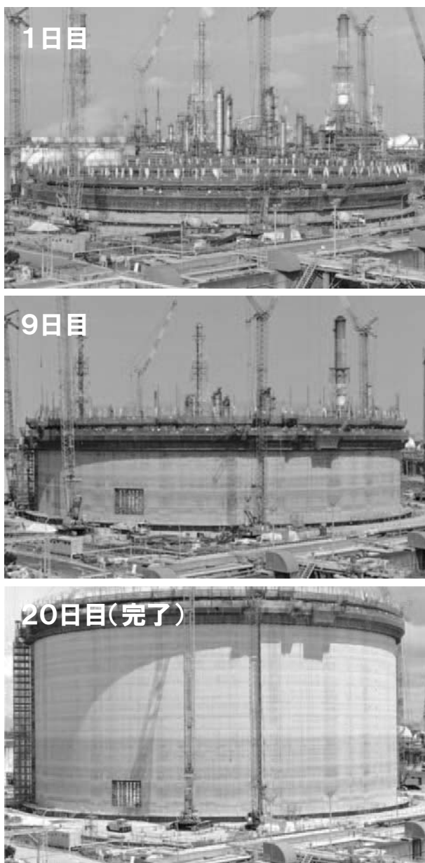
Fig. 14 Result of slipforming construction
