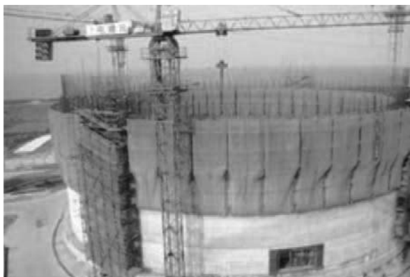
Fig. 6 Jumping form method of outer wall in China
