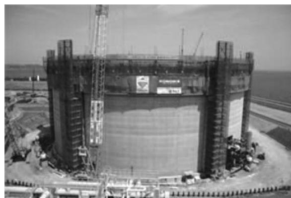
Fig. 7 Self-Climbing form method at Himeji, Japan
