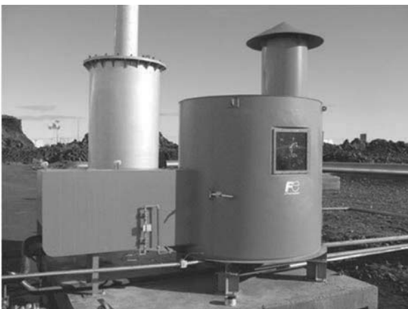
Fig. 9 Material test equipment at geothermal site
