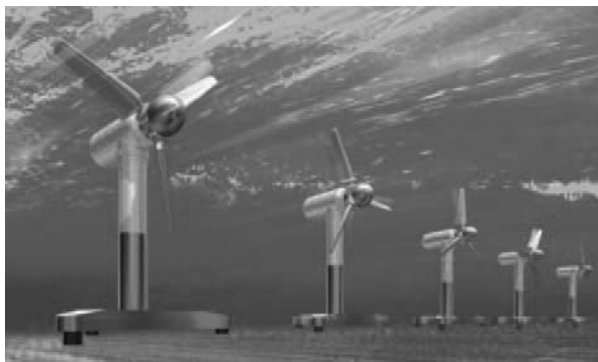
Fig. 2 Tidal turbine farm installed on seafloor (5)
