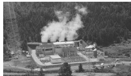
Fig. 1 The overall view of geothermal power plant (Mexico)
