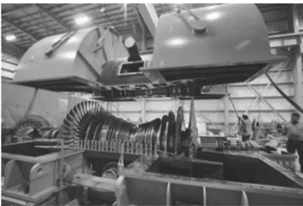
Fig. 15 Installation of 147MW turbine
