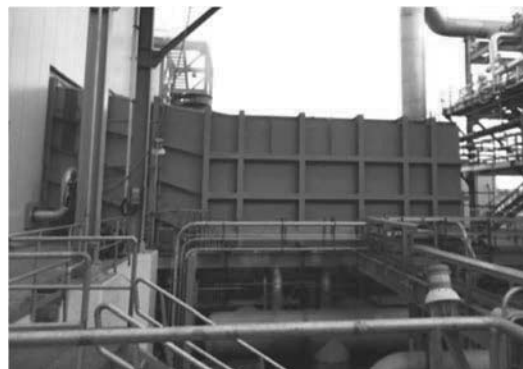
Fig. 12 The externals of direct contact condenser
