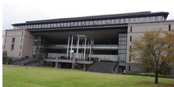
Fig. 3 Kagoshima Prefectural Citizens Exchange Center
