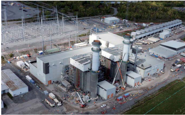
Fig. 10 Combined cycle power plant with M501GAC FAST
