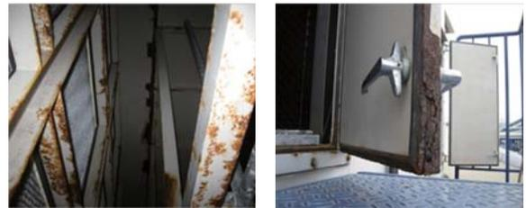
Fig. 32 Rust around the intake air filter box
