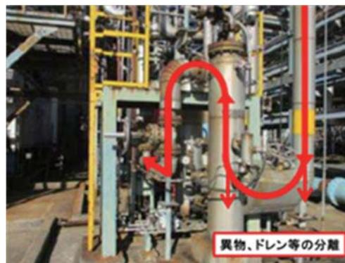
Fig. 10 Enhancement of drain collection
