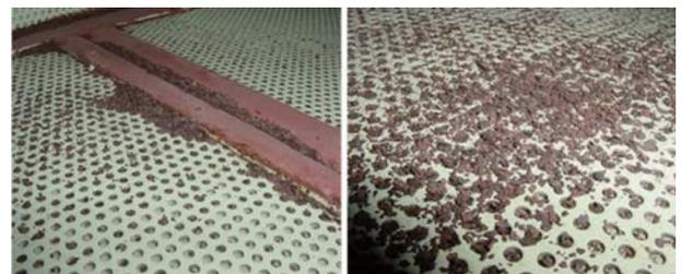
Fig. 33 Rust generated from inside the intake duct
