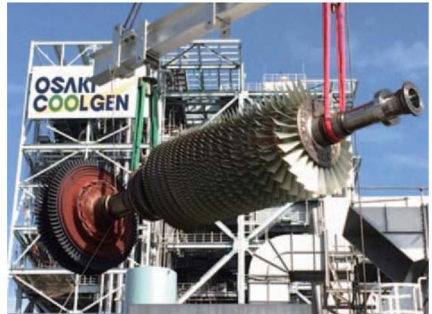
Fig. 15 (a) Lifting HP gas turbine
