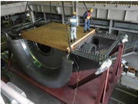
Fig. 14 Installation of new inner casing II
