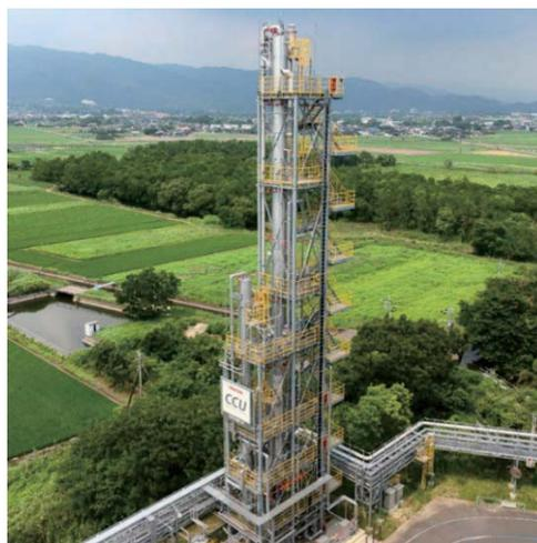
Fig. 7 CO<sub>2</sub> capture plant at Saga waste incineration plant
