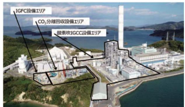
Fig. 8 Layout of demonstration test facilities
