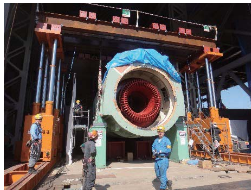
Fig. 16 Stator frame assembly by PJS
