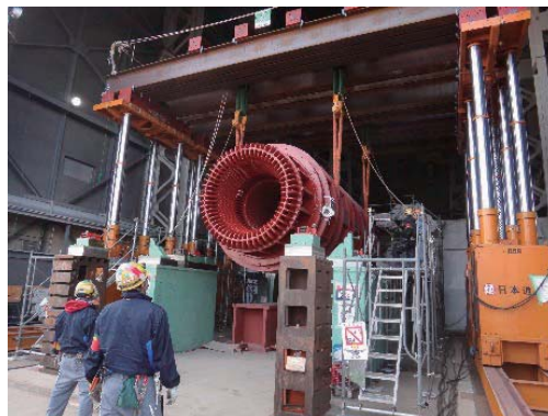
Fig. 15 Stator hoisting by PJS
