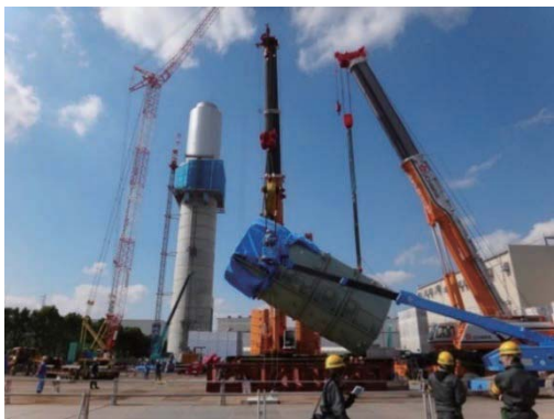
Fig. 12 Overturn stator frame by two cranes
