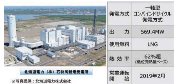
Fig. 3 Hokkaido Electric Power Company Ishikariwan Shinko Power Plant Unit 1
