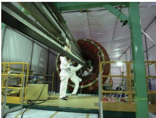
Fig. 14 Stator coil assembly by hanging tool
