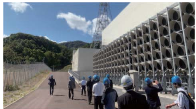
Fig. 10 Kita-Hon power grid connection facility (tour)
