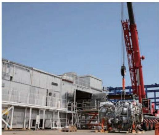
Fig. 6 SGT-750 core engine exchange (off-shore application)
