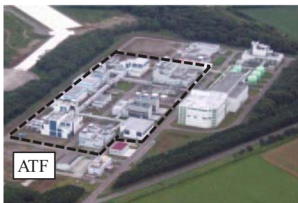
Fig. 4 ATF at Chitose Test Center, ATLA
