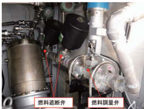
Fig. 2 Ammonia supply unit in the package
