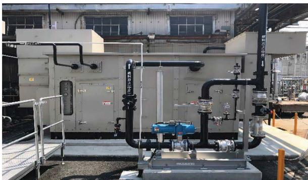
Fig. 6 Air-cooled gas compressor package
