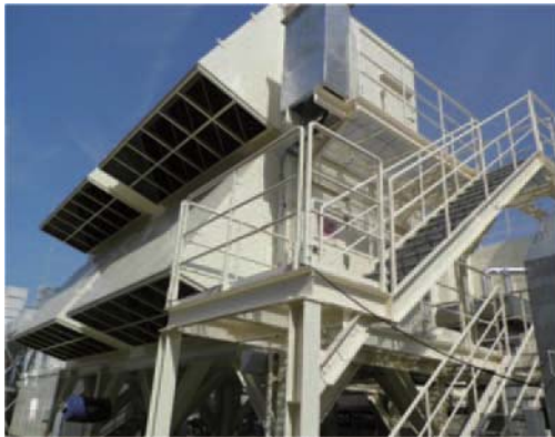
Fig. 12 Sample of GT intake filter house (2)
