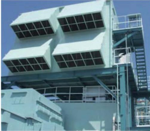
Fig. 11 Sample of GT intake filter house (1)
