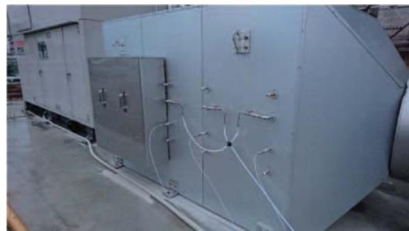
Fig. 6 NOx removal unit (SCR)
