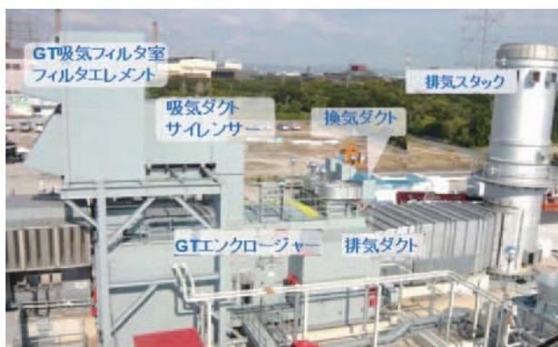
Fig. 10 Sample appearance of the whole GT package and our handled equipment
