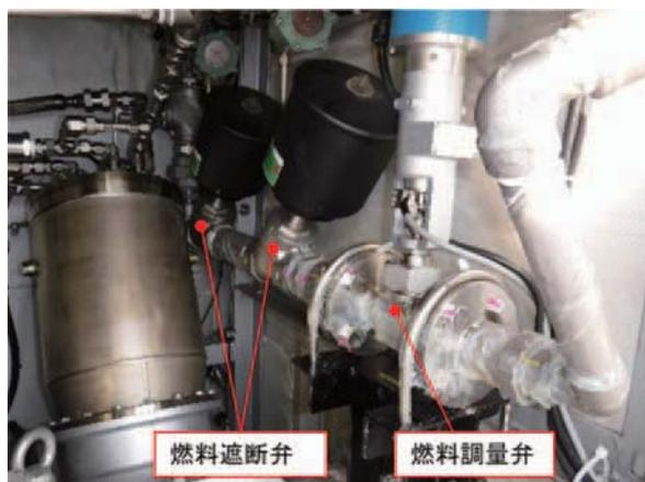
Fig. 2 Ammonia supply unit in the package
