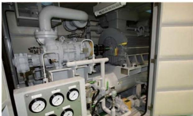
Fig. 2 Gas compressor unit (model 160M)
