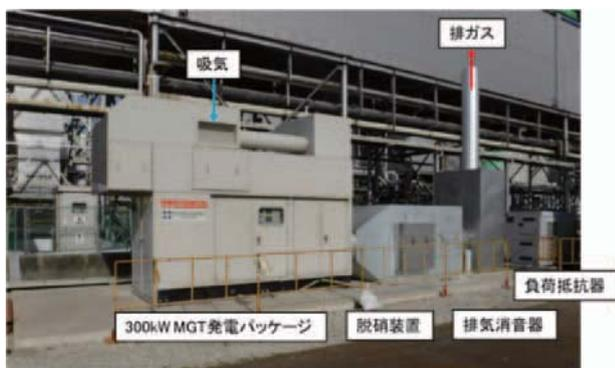
Fig. 1 300 kW ammonia combustion MGT package
