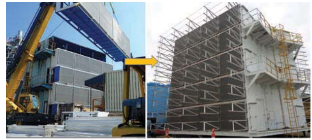
Fig. 15 Rehabilitation of GT intake filter house
