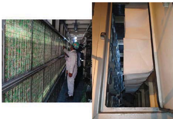
Fig. 9 Photo of modification working in filter house
