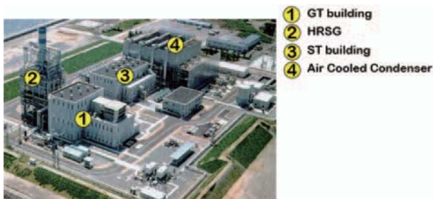
Fig. 3 Gas turbine combined cycle power plant (Validation facility) in takasago factory
