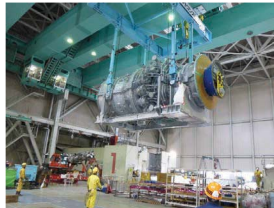
Fig. 2 Gas turbine upgrade work at Kawagoe Power Plant (Gas turbine installation)
