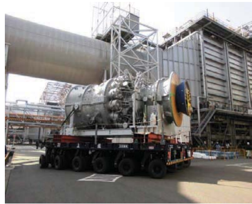
Fig. 1 Gas turbine upgrade work at Kawagoe Power Plant (On-site transportation)
