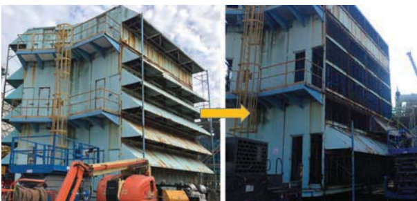
Fig. 14 Rehabilitation of GT intake filter house
