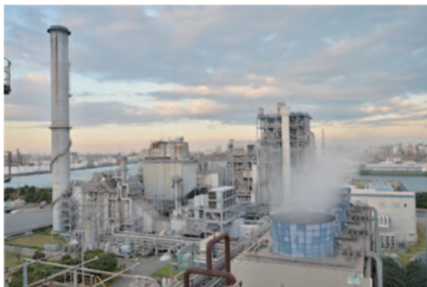
Fig. 13 Mizue thermal power plant of TOA OIL CO., LTD
