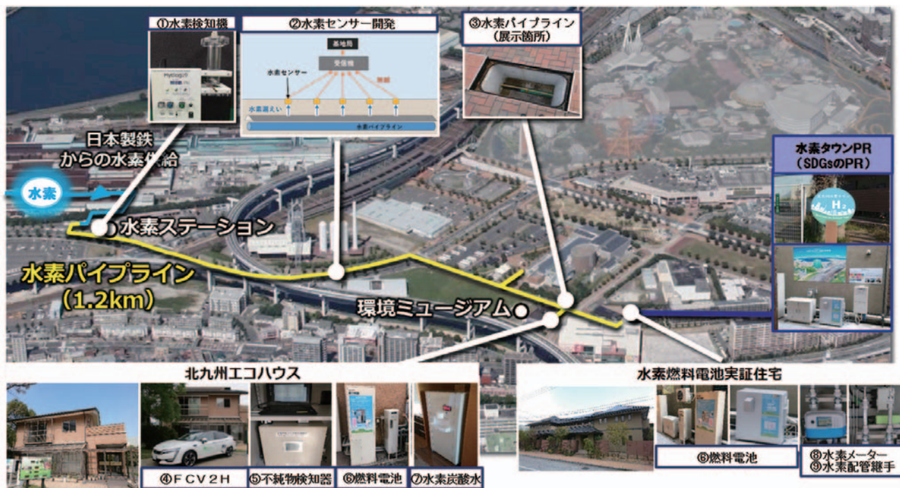
Fig. 10 Pipeline installed in Kitakyushu Hydrogen Town
