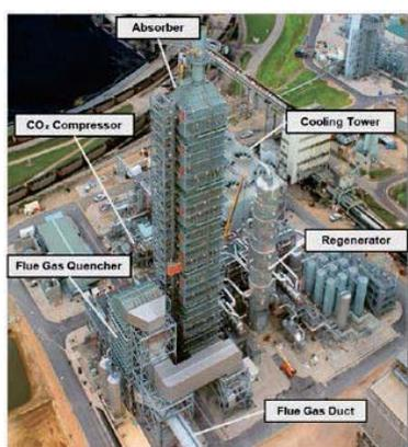
Fig. 13 World's largest CO<sub>2</sub> recovery plant
