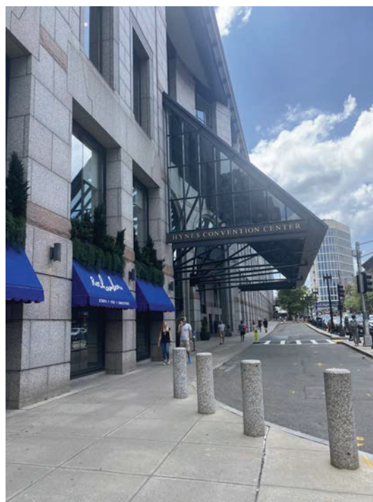
Fig. 1 A View of the Hynes Convention Center from Newbury Street.
