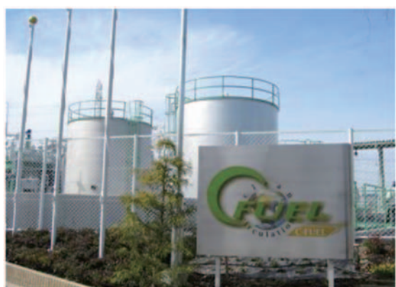
Fig. 5 C-FUEL manufacturing plant
