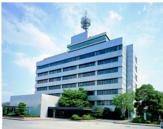
Fig. 1 Fundamental Technology Research Institute of Toho Gas Co. Ltd.
