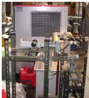
Fig. 5 Micro Gas Turbine
