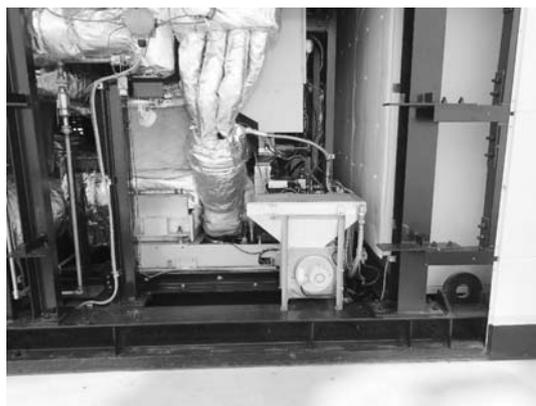
Fig. 13 MGT installed in SOFC
