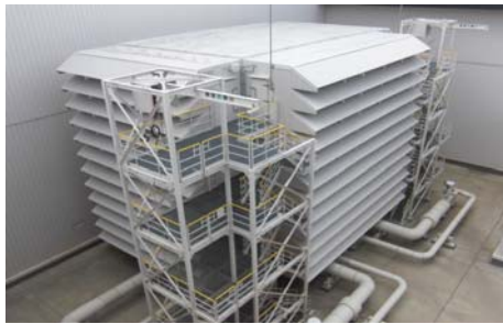
Fig.5 Snow Protection Hoods and Anti-icing System
