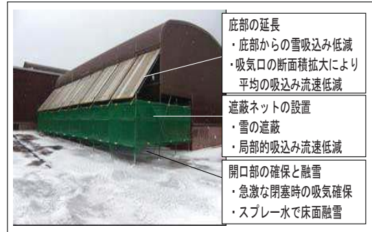
Fig.4 Applications at the Air Intake to Prevent the Inlet Air Filter Clogging by the Snow
