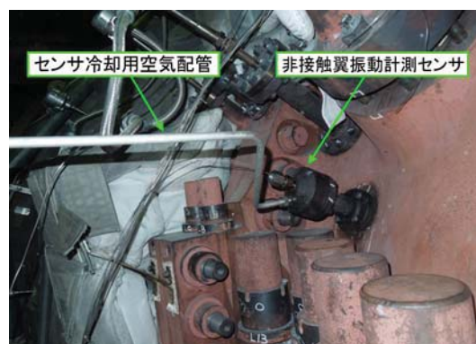
Fig.13 Non-contact blade vibration measurement using an actual gas turbine of gas turbine blade under actual operating condition
