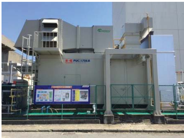
Fig.3 Overview of demonstration plant
