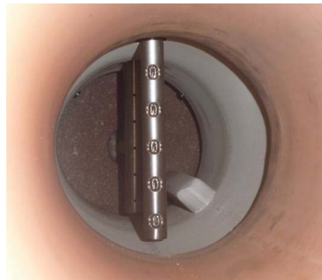
Fig.8 Temperature probe and gas sampling probe mounted inside exhaust duct
