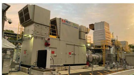
Fig.2 Picture of hydrogen fueled gas turbine co-generation power plant (1MW class gas turbine package, HRSG)
