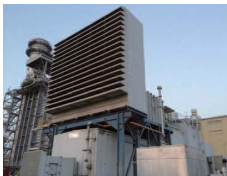
Fig. 8 Sample appearance of GT air intake filter house which contains Cartridge type filter
