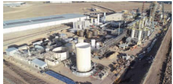
Fig. 4 Fulcrum's SAF Production Plant under Construction (as of Dec 2020)
